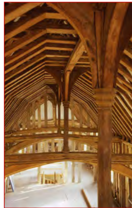
The Great Hall roof
